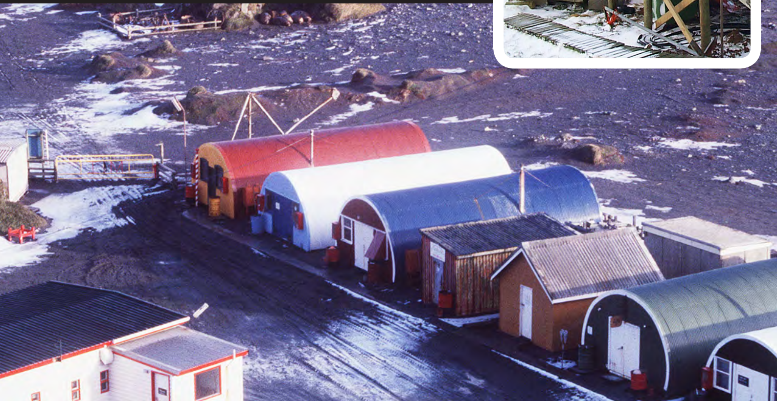
Images - Right: Field hut at Brothers Point, Macquarie Island, 1999. Photographer Dale Main. Below: (L-R) Plumbers workshop, field store, carpenter, Hardware store, Sealers Inn and Electrical workshop, 1987. Photographer Mark Loveridge.
