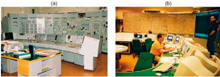
FIG. V-4. (a) Sweden's Oskarshamn unit 1 MCR before modernization in 2003; (b) after modernization.
