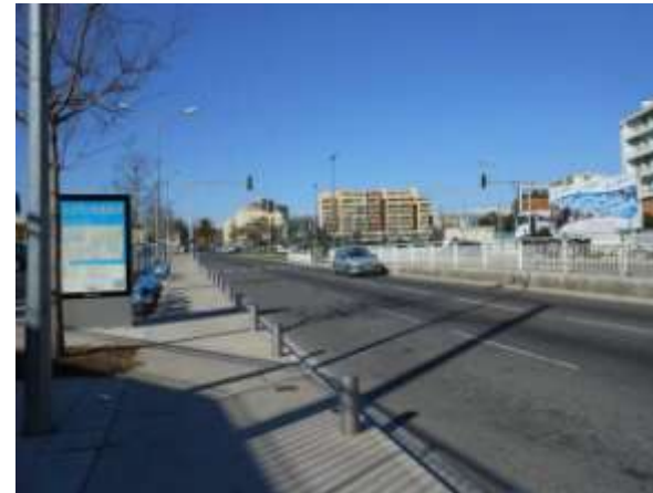
Photo Egis France
