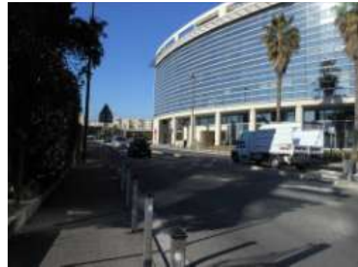
Photo Egis France
