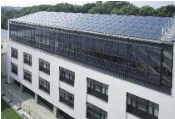
grid-connected BIPV system on the roof and façade of a commercial building.
