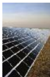
Large Thin Film power plant.
