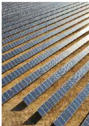
Large ground-mounted PV plant, Mallorca, Spain.
