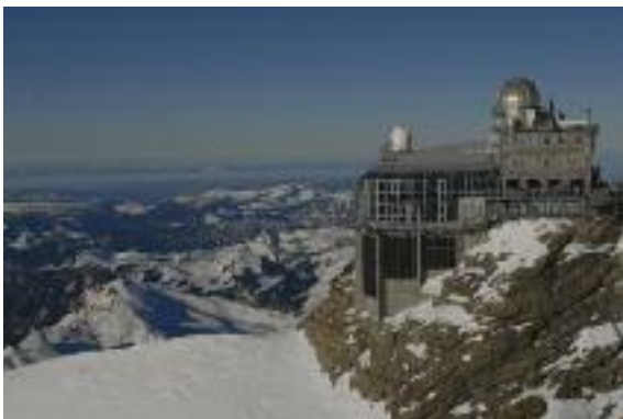
Off-grid industrial application.
