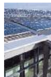
PV modules integrated into flat roof.
