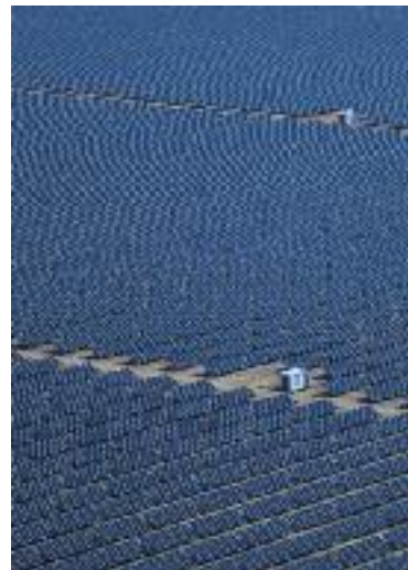
Large ground-mounted PV system in Spain.
