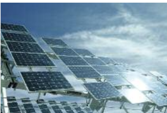
PV power plant in Darro, Spain.
