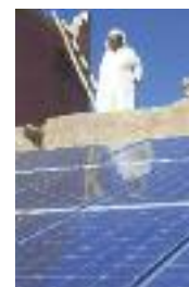
Off-grid PV system in Morocco.
