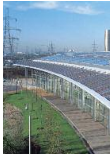
PV system integrated on a roof.
