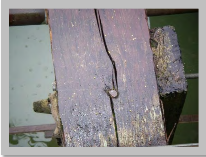
Figure 6.9: The connection on this pier in the CEI Hub appears to have deteriorated due to a split in the timber beam. This type of damage suggests that the condition of the structure may not be routinely monitored and maintained and that the overall pier is seismically vulnerable (Source: DOGAMI photo)
