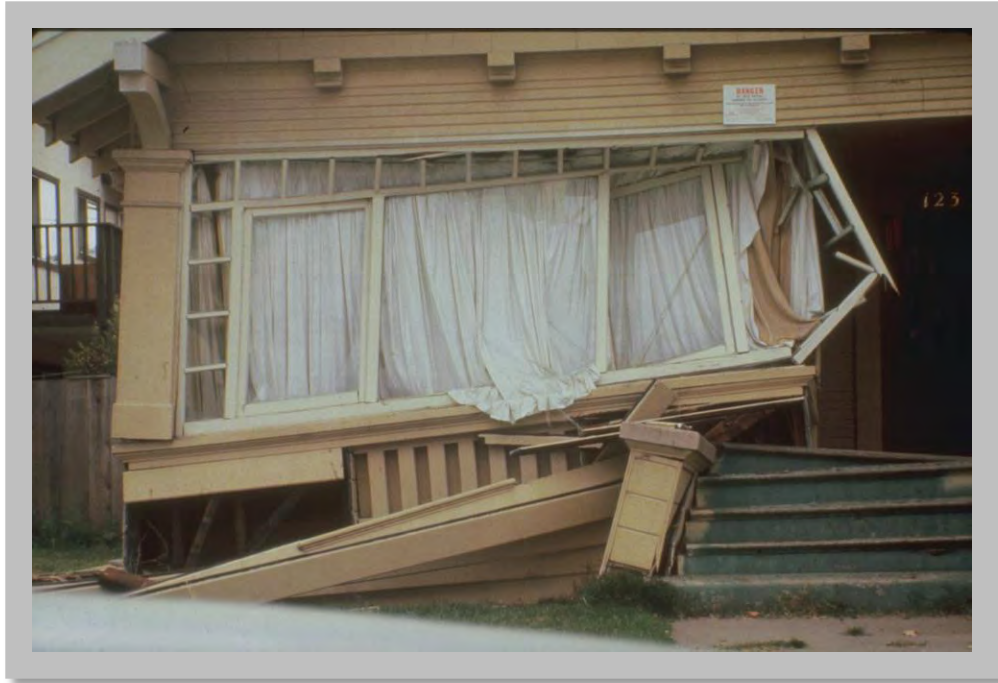
Figure 4.8: This residential building shifted on its foundation after the 1989 M 7.1 Loma Prieta, California earthquake. (Source: NOAA/NGDC, C. Stover, U.S. Geological Survey)
