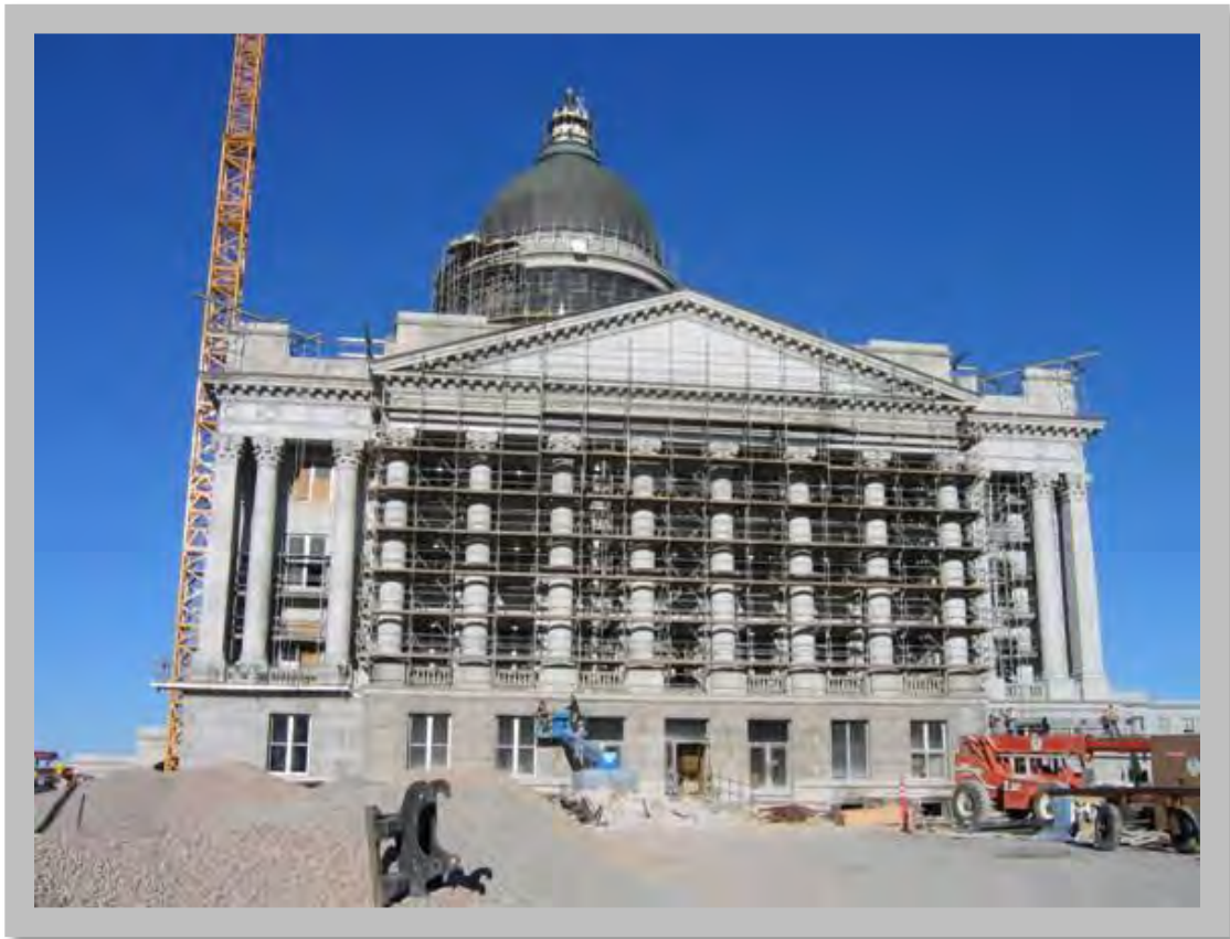
Figure 4.7: Several states have rehabilitated their state capitol buildings. The Utah State Capitol was seismically retrofitted with base isolation to protect visitors and occupants and preserve historic fabric in the building. (Source: State of Utah)
