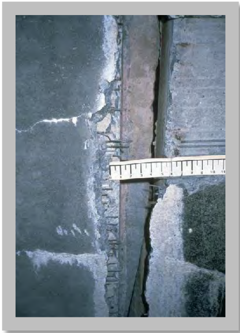
Figure 8.3: Wire wrapped concrete tank burst in Purisima Hills, Loma Prieta earthquake, California, 1989 (Source: Photo by Don Ballantyne)
