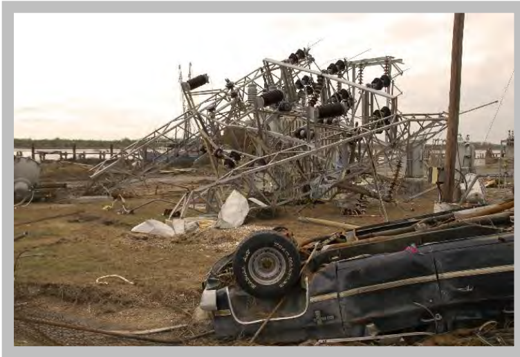
Figure 3.4: Hurricane Katrina Storm Surge – Electric Facility. Replacement of coastal power infrastructure based on 2012 capabilities may take one to three years for the Earthquake-only zone. (Source: FEMA.gov)
