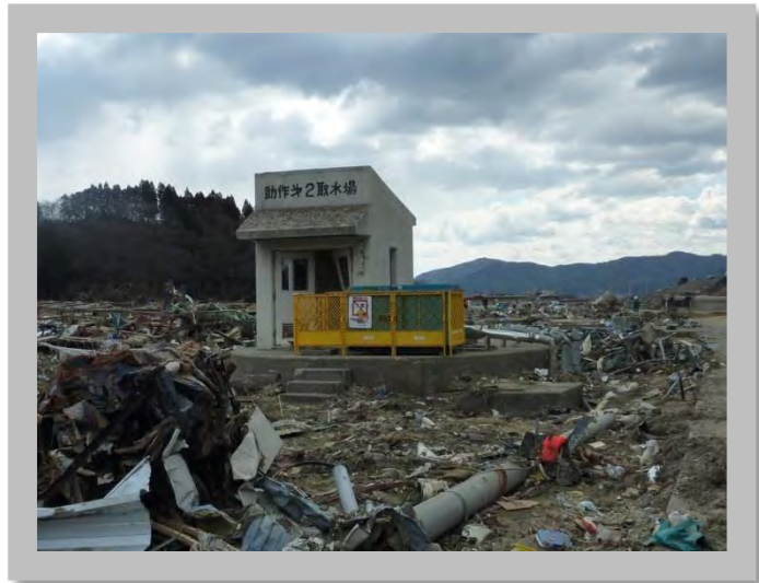
Figure 8.6: Water well and treatment facility in tsunami inundation area, Tohoku earthquake, Japan, 2011 (Source: Photo Source Unknown)
