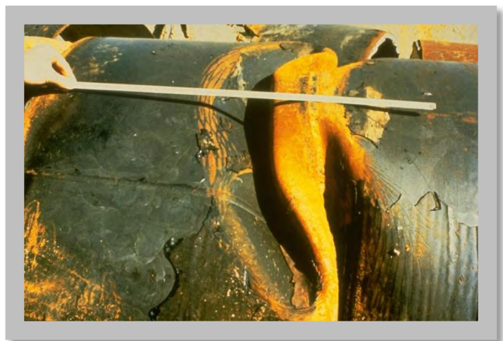
Figure 8.4: Welded steel pipe failed in compression, San Fernando (Sylmar) earthquake, California, 1971 (Source: Photo Source Unknown)
