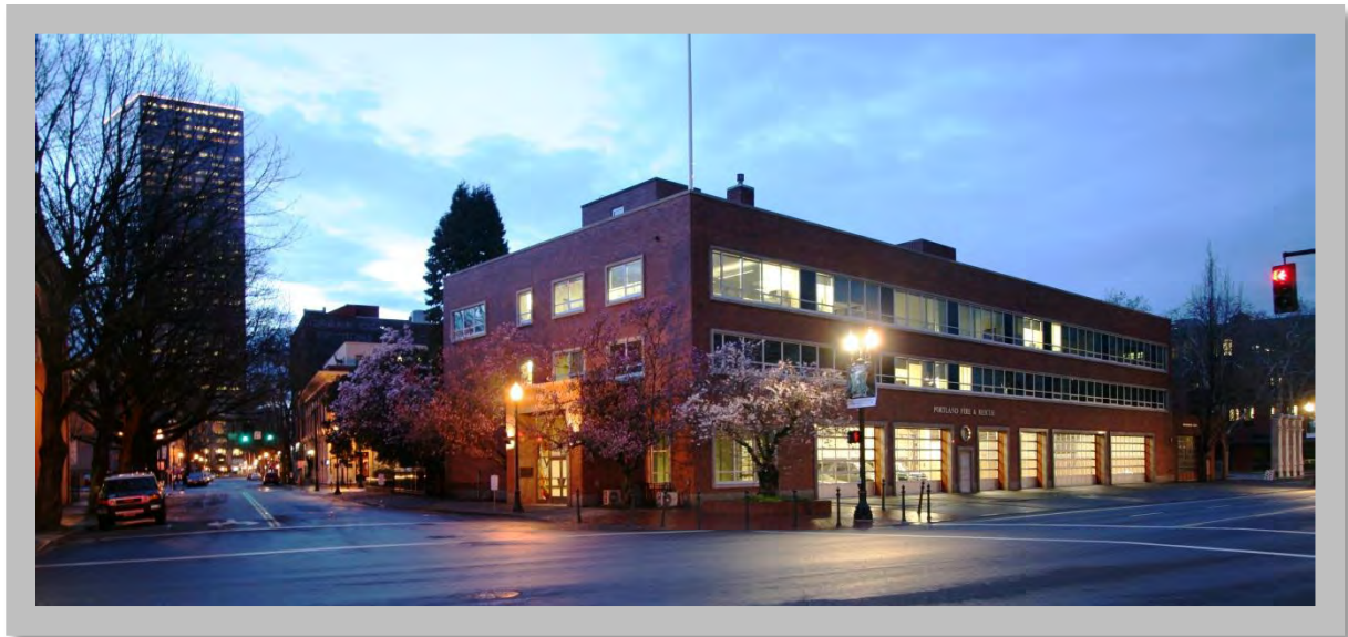
Figure 4.4: Some cities in Oregon have already started seismic rehabilitation program to strengthen the fire stations that are susceptible to serious damage in an earthquake. Fire Station #1, the largest in Portland, was retrofitted in 2009. It should now be in working order after an earthquake, serving downtown Portland. (Source: Peck Smiley Ettlin Architects)
