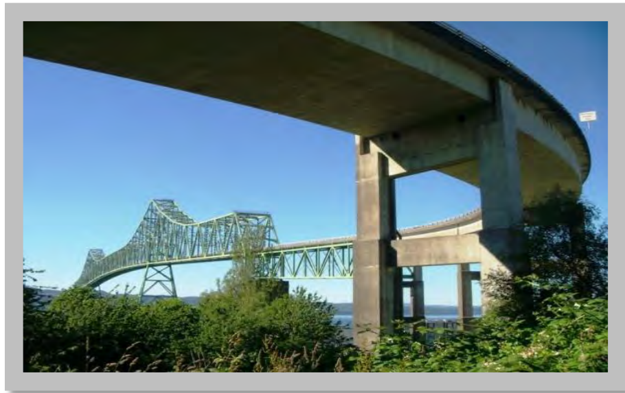
Figure 6.10: The approach (foreground) to the 1966 Astoria-Megler Bridge that spans the Columbia River has major structural deficiencies that could lead to a collapse following an earthquake. Damaged bridge sections could block waterway access to the CEI Hub. (DOGAMI photo)
