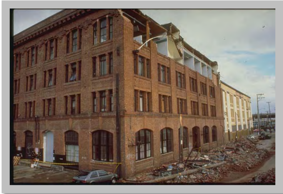
Figure 4.11: The fourth-story wall of this unreinforced masonry building on Bluxome Street in San Francisco collapsed onto the street, killing five people in their cars, during the M7.1 October 18, 1989 Loma Prieta, California earthquake. (Source: NOAA/NGDC, E.V. Leyendecker, U.S. Geological Survey)
