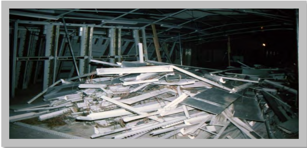
Figure 7.2: The overhead lighting fixtures in a Central Office failed during an earthquake. Note the equipment in the background was supported by “jiffy poles” after the earthquake. Mexico City earthquake, 1985. (Source: Alex Tang)
