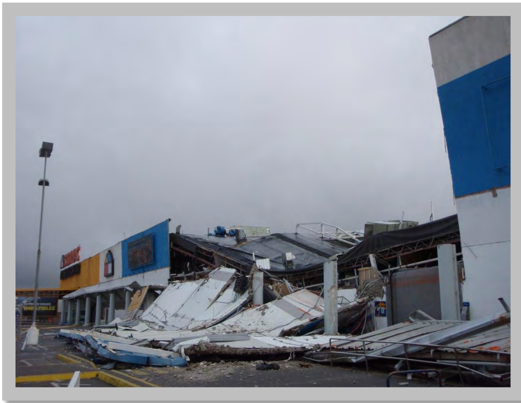
Figure 4.9: Several tilt-up concrete panels of this construction material supply store in Concepcion fell away from the building, causing the roof framing to collapse after the M 8.8 February 27, 2010 Maule Chile earthquake. (Source: Kent Yu, Degenkolb Engineers)
