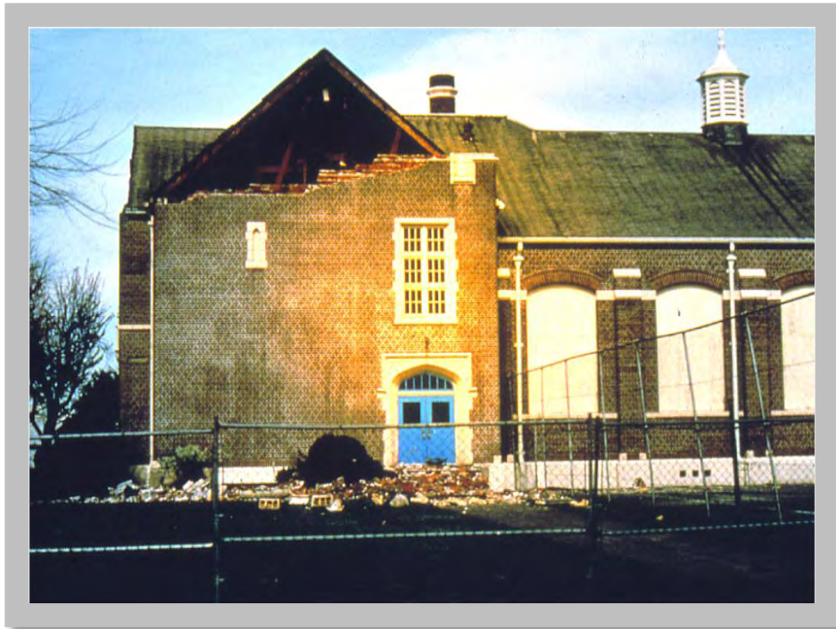
Figure 4.5: The previous Molalla High School building, a three-story unreinforced masonry structure, was damaged from the M5 .6 Scotts Mills, Oregon earthquake in 1993. It happened during spring break, when the school was empty, which prevented serious injuries. The district took the opportunity to forecast future needs and decided not to rebuild at the same location. Molalla High School is now housed on a larger campus with a stronger, more spacious building. Many URM schools and other buildings in Oregon could suffer a similar fate in future earthquakes. Communities can act now to plan how and when to rehabilitate or replace these aging, potentially dangerous facilities. (Source: DOGAMI)
