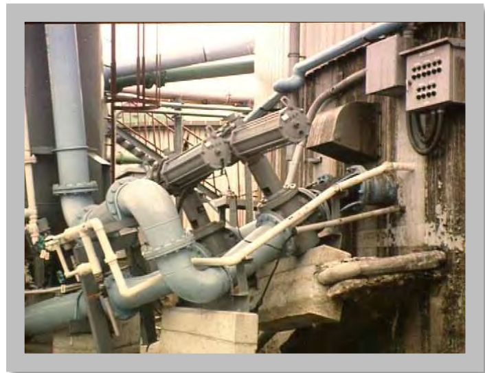
Figure 8.15: Damage from liquefaction/lateral spreading at Higashinada WWTP, Kobe, Japan, 1995 (Source: Photo by Don Ballantyne)
