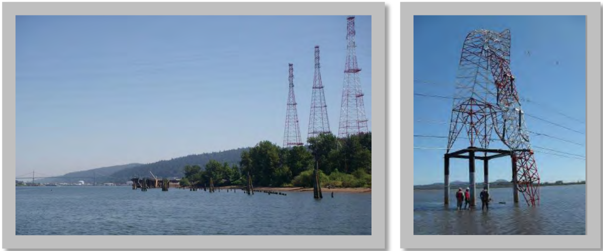
Left: These high voltage electrical transmission towers are built on a river bank in the Critical Energy Infrastructure (CEI) Hub susceptible to lateral spreading. (DOGAMI photo) Right: Structural damage to a high voltage transmission tower located at a river crossing in 2010 Chile earthquake (ASCE Technical Council on Lifeline Earthquake Engineering – TCLEE)
