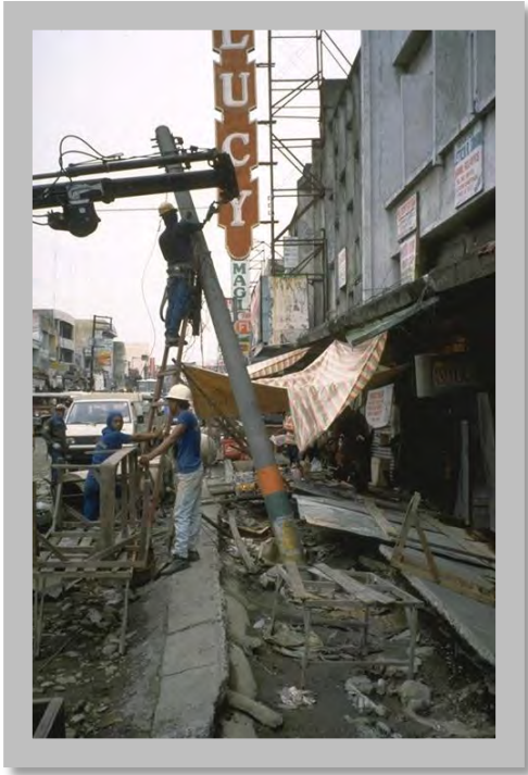
Figure 8.16: Sewer line that floated to the surface as a result of liquefaction, Dagupan, Philippines, 1990. (Source: Photo by Don Ballantyne)
