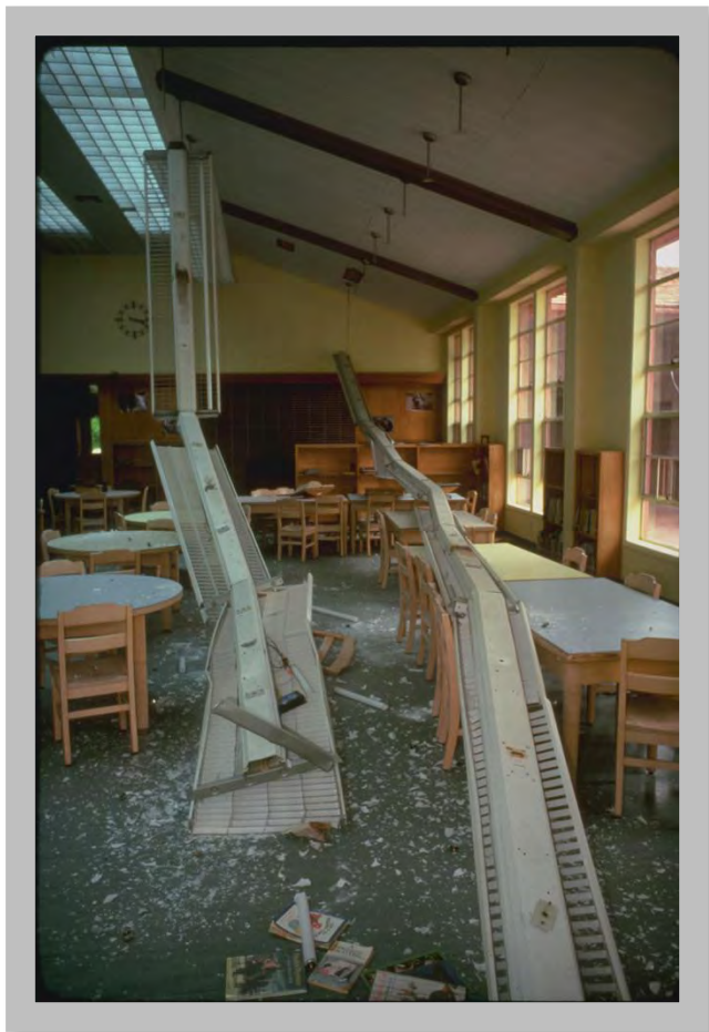
Figure 4.6: Pendant light fixtures failed in this elementary school library during the 1983 M6.5 Coalinga, California earthquake. If the room had been occupied, this could have caused injuries. Bracing nonstructural elements in homes, schools, and offices can often be done easily and relatively inexpensively. (Source: NOAA/NGDC, Earthquake Engineering Research Institute)
