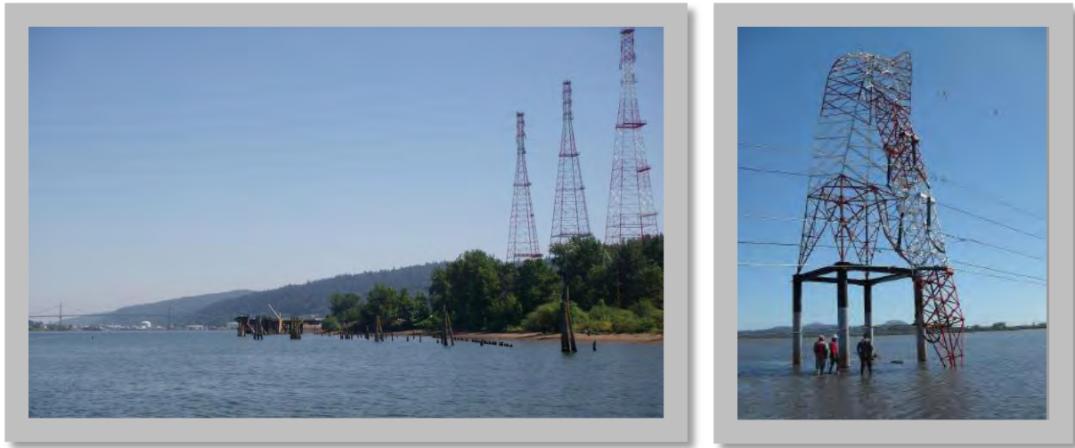
Figure 6.11 and 6.12: Left: These high voltage electrical transmission towers are built on a river bank in the CEI Hub susceptible to lateral spreading. (DOGAMI photo) Right: Structural damage to a high voltage transmission tower located at a river crossing in 2010 Chile earthquake. (ASCE Technical Council on Lifeline Earthquake Engineering – TCLEE)
