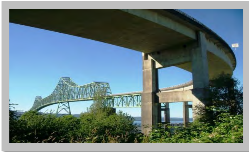
The approach (foreground) to the 1966 Astoria-Megler Bridge that spans the Columbia River has major structural deficiencies that could lead to a collapse following an earthquake. Damaged bridge sections could block waterway access to the Critical Energy Infrastructure Hub. (DOGAMI photo)
