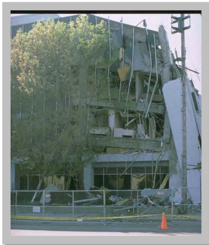
Figure 4.12: This non-ductile concrete frame medical building collapsed during the 1994 M6.8 Northridge, California earthquake. (Source: NOAA/NGDC, J. Dewey, U.S. Geological Survey)
