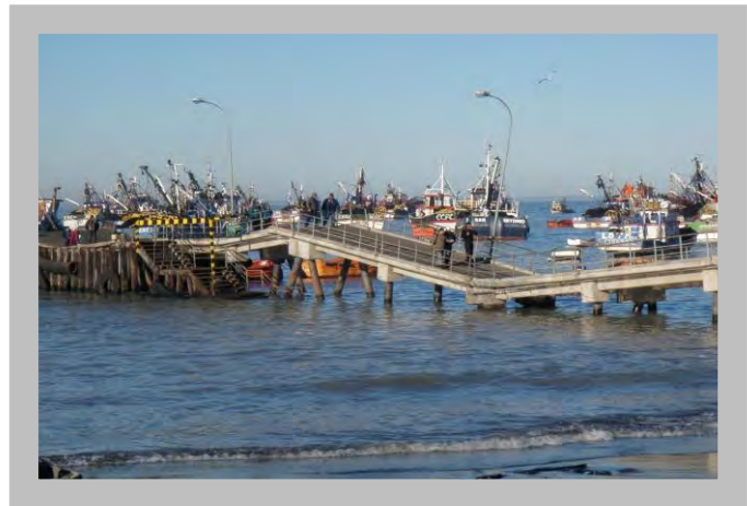
Figure 6.6: An example of a damaged pier in the 2010 Chile earthquake (ASCE Technical Council on Lifeline Earthquake Engineering – TCLEE, 2010)
