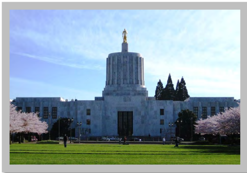
Many of existing public and private buildings such as the State Capitol Building were built prior to our knowledge of the Cascadia subduction earthquake. They are not seismically safe, and pose significant life-safety threat to the building occupants. Photo Source:
