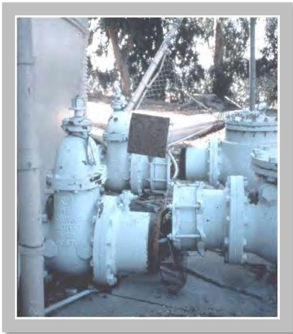
Figure 8.1: Tank piping separated, Northridge earthquake, California, 1994 (Source: Los Angeles Department of Water and Power)
