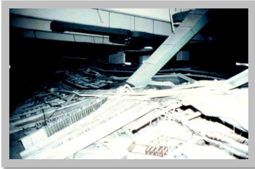
Figure 7.4: Telecom equipment and HVAC ducting failure. It is hard to tell which was the main cause of failure; it has several combinations, inadequate anchoring, un-braced duct supports, etc. Mexico City earthquake, 1985. (Source: Alex Tang)
