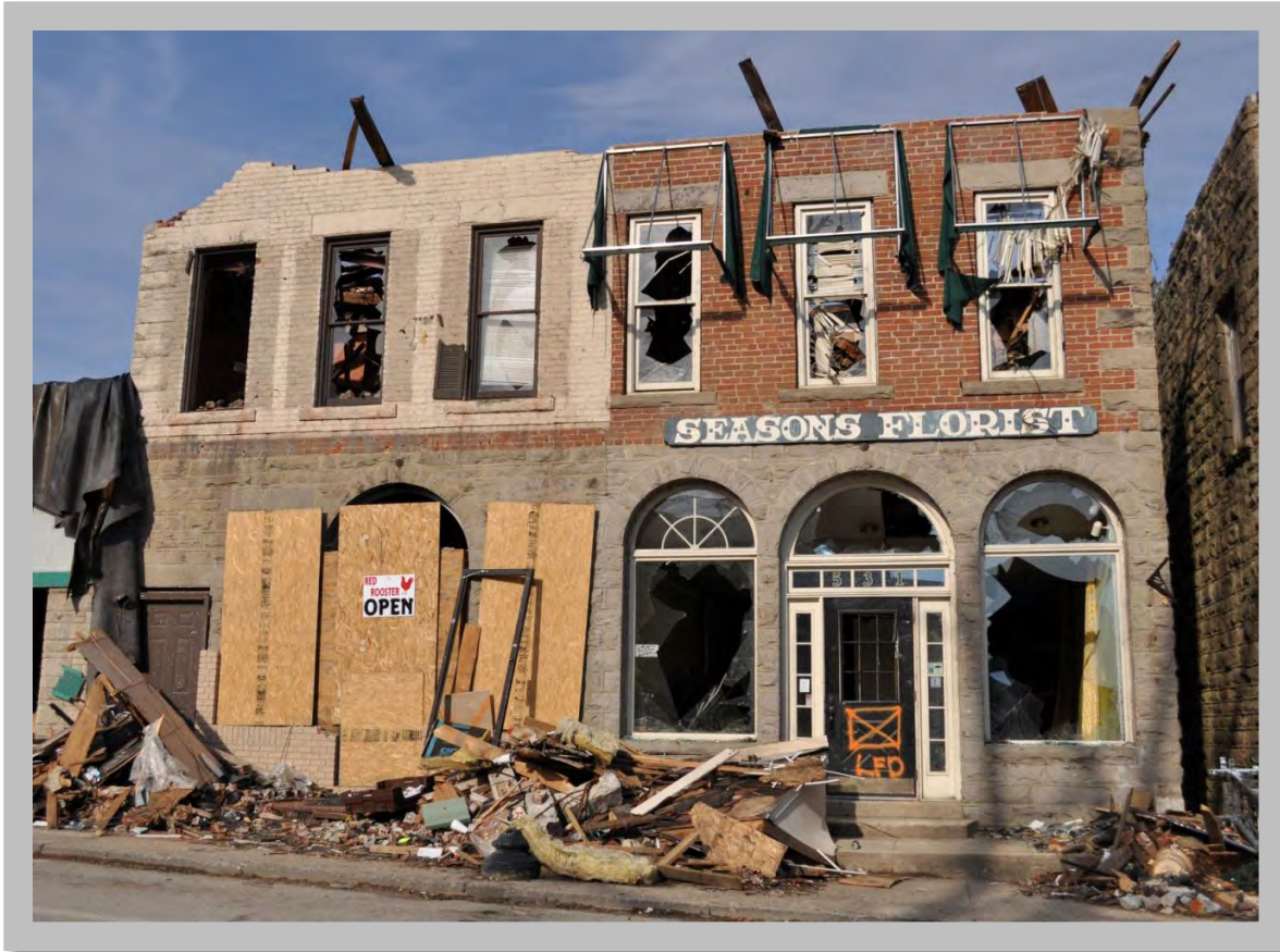
Figure 2.13: West Liberty, Ky., March 19, 2012 -- Destroyed buildings, many with historical significance, line the streets of downtown West Liberty. FEMA is working with Commonwealth and local officials to remove debris and demolish buildings that cannot be saved. (Source: Photo by Marilee Caliendo/FEMA)
